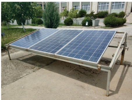
Fig. 1. Solar energy system installation
